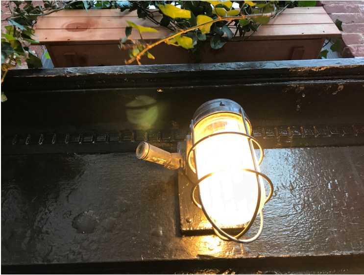
Closeup of light over main entry door
